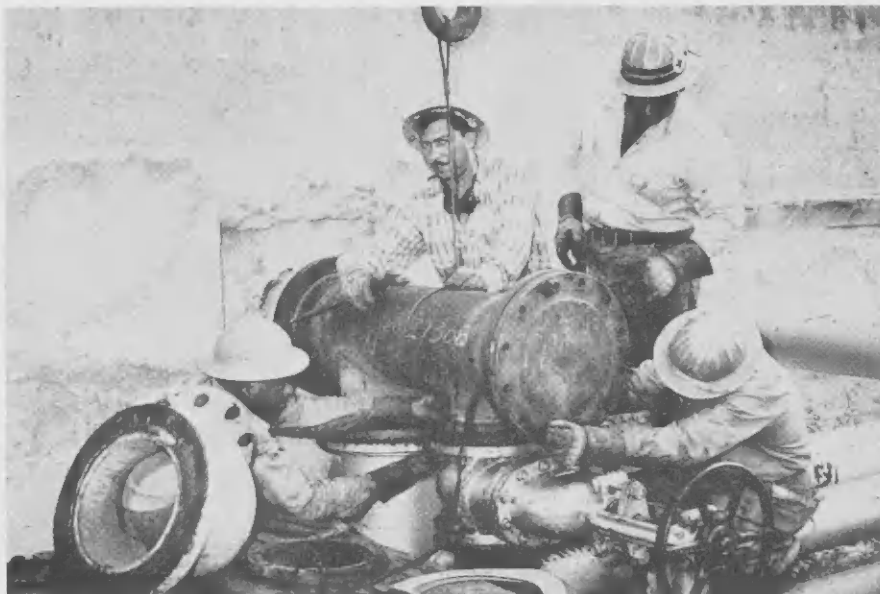
SOON AFTER his suggestion was accepted, Mechanical Department craftsmen began "hot tapping" the kerosine production line, left. PRONTO DESPUES cu su sugerencia a worde aceptá, hendenan di Mechanical Department a cuminsa cu « trabao di "hot tap" ariba e linja di kerosine, robez.
